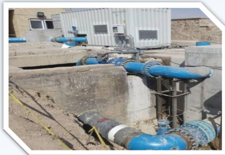
3 MW capacity Small Hydropower (Semnan Province, Iran)
