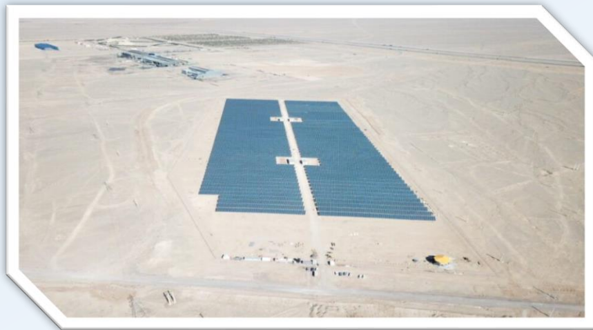
10 MW capacity PV power plant (Yazd Province, Iran)
